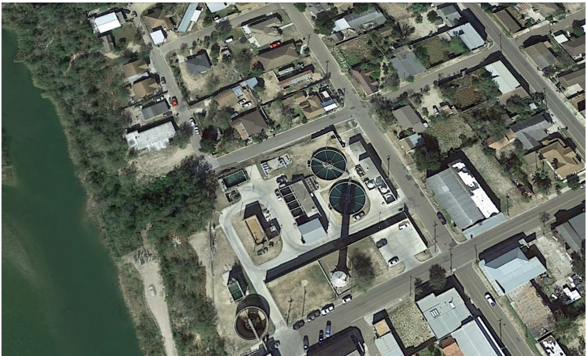
The City of Roma's Drinking Water Treatment Facility
