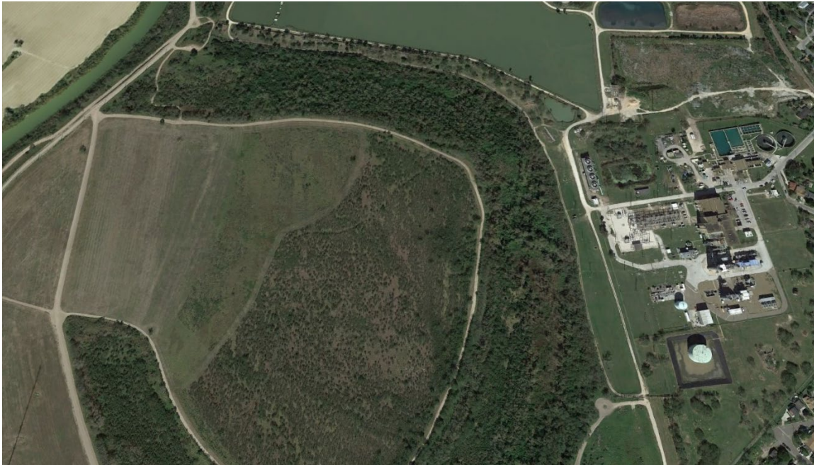
The Brownsville PUB's Silas Ray Power Plant
