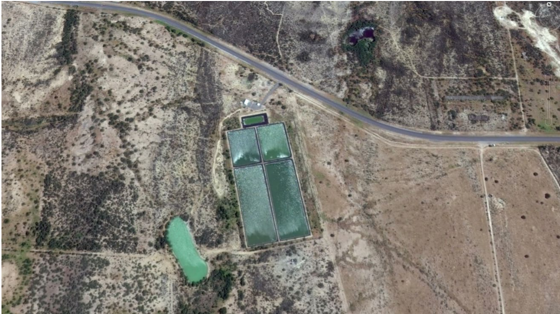
Ciudad Mier's Wastewater Treatment Facility
