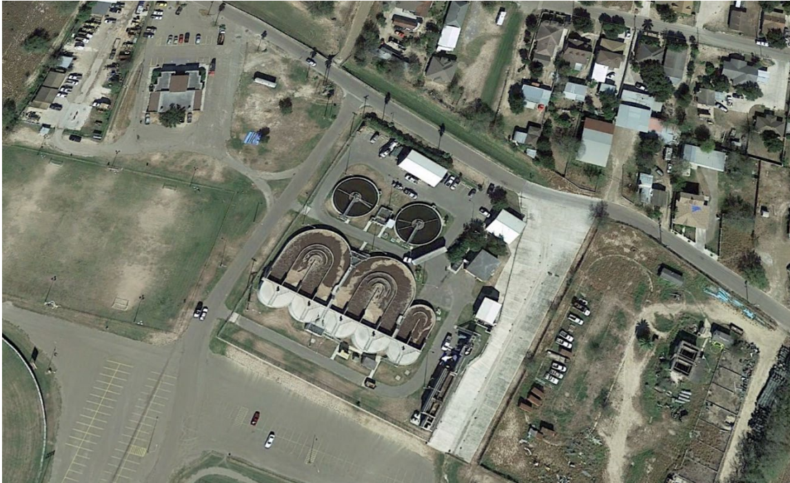
The City of Roma's Wastewater Treatment Facility
