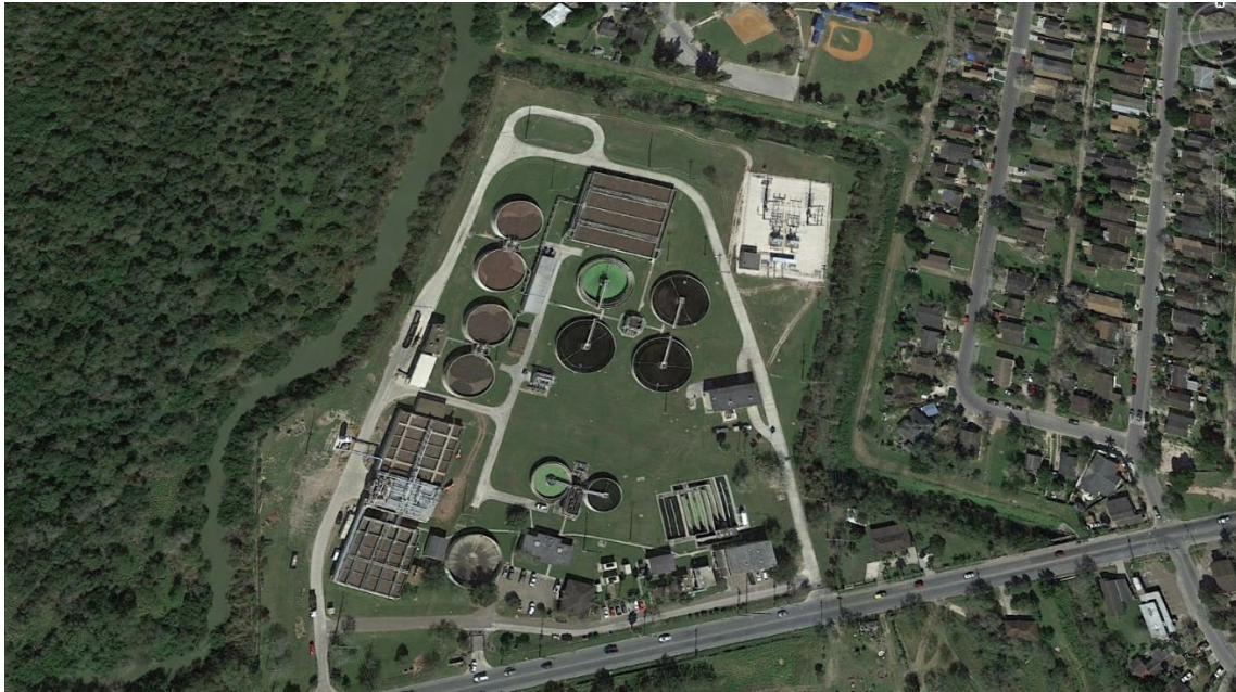
The Brownsville PUB's Southside Wastewater Treatment Facility
